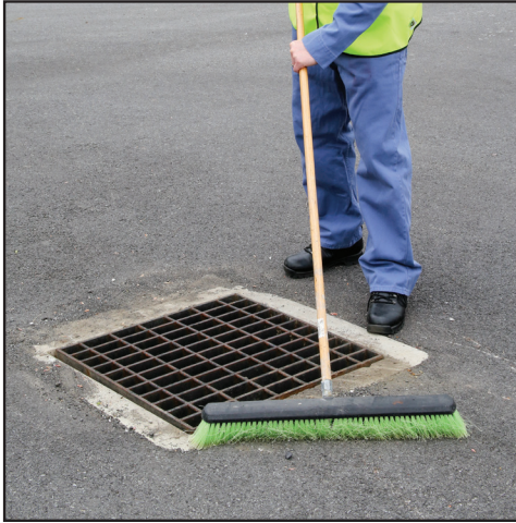
Step 1. Prepare surface around the drain, making sure it's free of debris.
